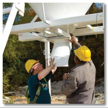
Install the slide gate assembly under the silo.
