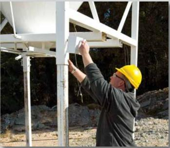
**2** After placing the silo on the ground at the desired job site location, remove the silo leg pins.
