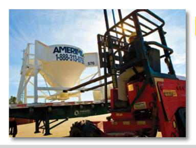
Using the silo's welded forklift tubes, offload the silo from the truck using a forklift.
