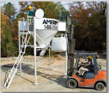
Using the bulk bag's nylon straps, lift the bag into place with the forklift and position above the silo's charge hatch. Unzip the bottom of the bag. A spout will drop down allowing the dry material to be unloaded into the silo.
